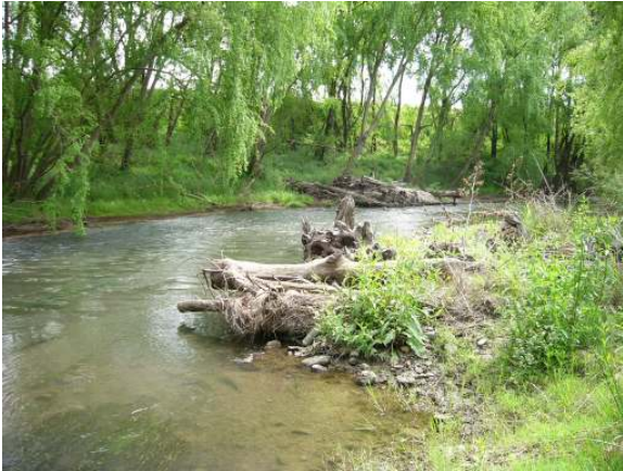
Engineered log jams at the 'Fish Riffles' site on the Hunter River.
