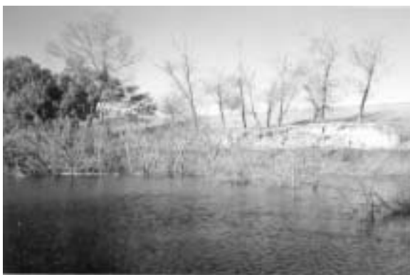
An example of streambank erosion along the Hunter River. Extensive land clearing along streambanks has made this a common sight.
