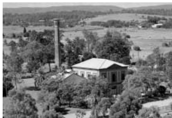
Walka Water Works (Oakhampton) was built in 1887 to supply domestic water to Newcastle and the Lower Hunter.
