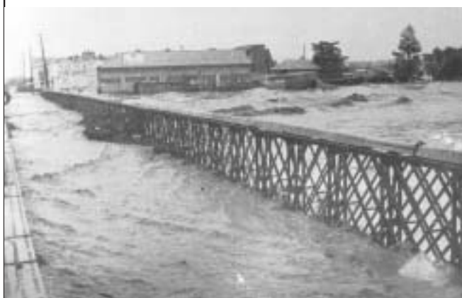
Tearing of the 1955 floodwaters at the old Belmore Bridge, taken from Lorn looking back towards the Courthouse and High Street.
