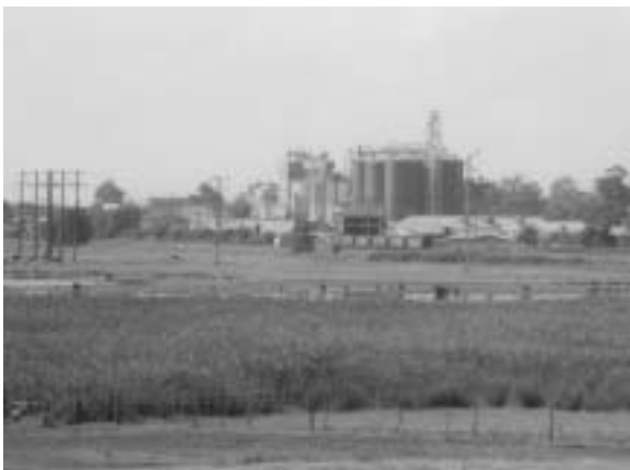
Steggles has a licence to discharge waste waters to the swamp but has embarked on a process to reduce the volume of discharge (e.g. through improved water efficiency and alternative uses of waste water).
