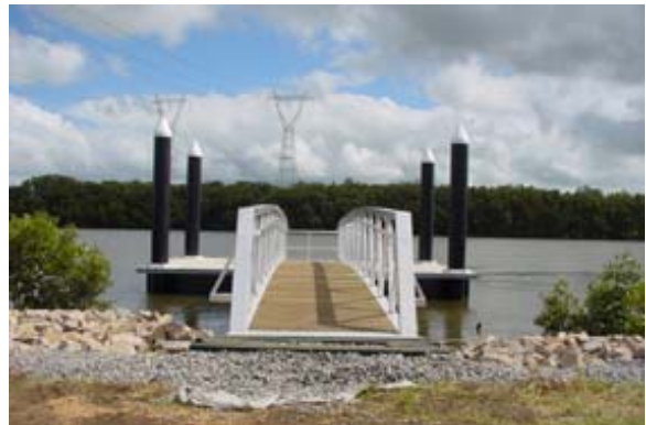
City Farm Jetty, linking land and river visitation and adding to the amenities of the North Arm of the Hunter River.
